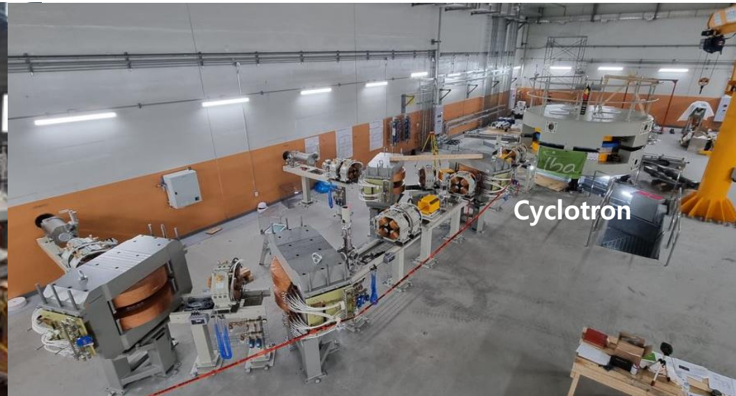
Cyclotron beam line installation
